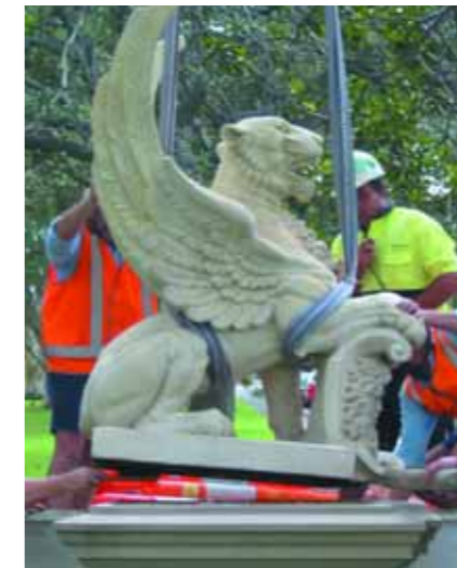
Carefully installing the griffins
