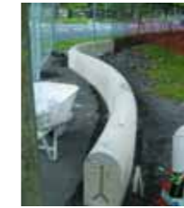
Jervois Gates under repair
