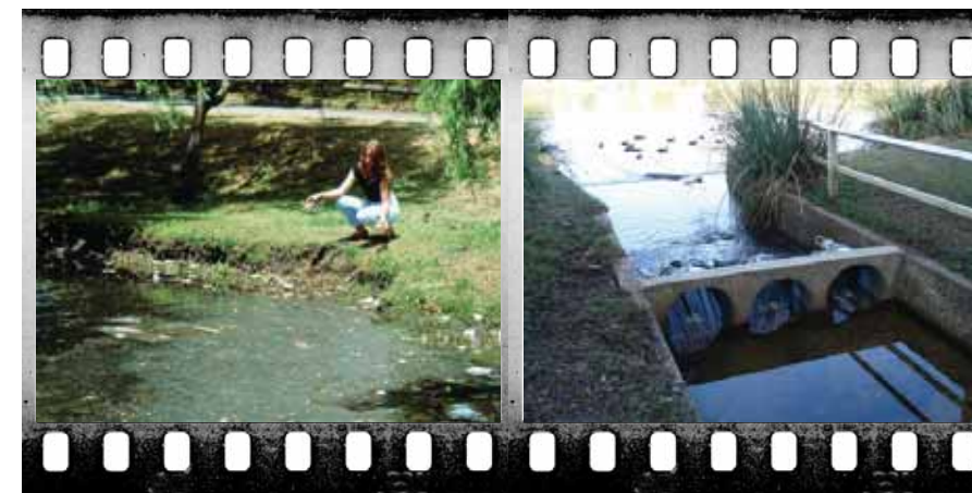
Rubbish in Centennial Parklands ponds was a big problem in the 1980s, however the installation of Gross Pollutant Traps, among other measures, has contributed to curtailing rubbish in the ponds.
