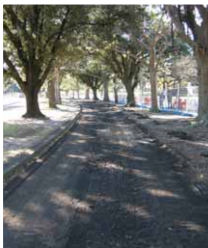
Works in progress on Grand Drive footpaths"
