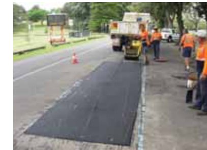
Grand Drive patching work in action
