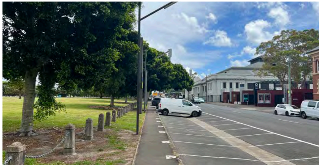
Existing condition of Driver Avenue
